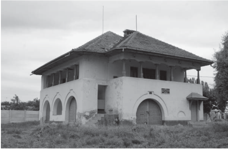
Figure 2. A boyars' house, at present kindergarten (photo by Gabriela Boangiu)
