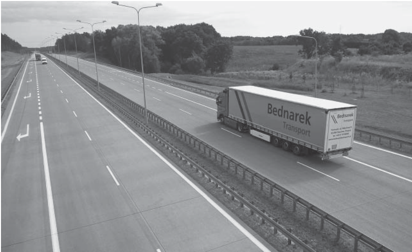
Figure 1. Motorway A2, Torzym, Lubusz Voivodeship, 2015 (photo by Waldemar Kuligowski)
