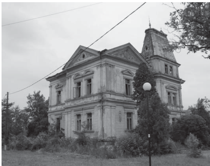
Figure 1. The mansion of Poenaru family from Malu Mare, former high-school of the commune in the communist period (photo by Gabriela Boangiu)
